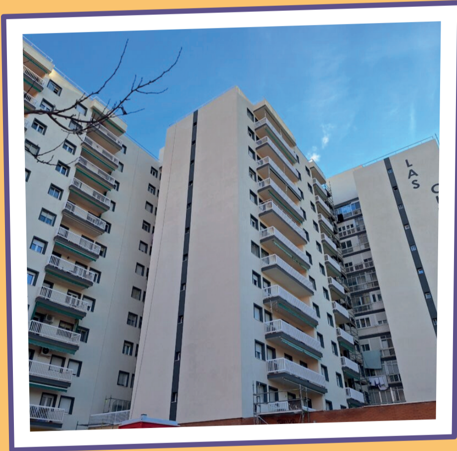
Guadalajara, Spain Multifamily and multi floor residential building
