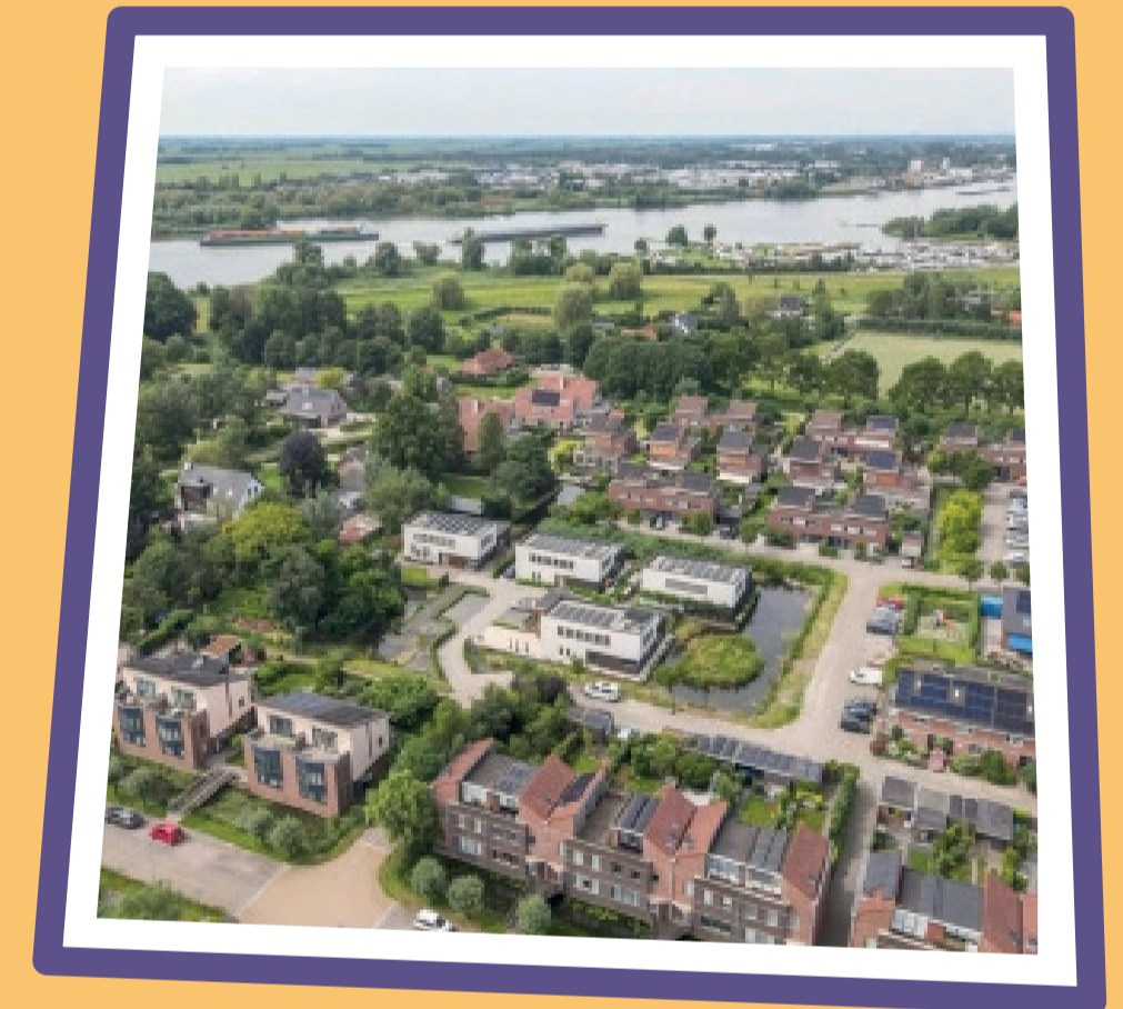
Watervliet, The Netherlands Energy-positive homes combining PV, batteries, heat pumps and EMS to reduce grid congestion.
